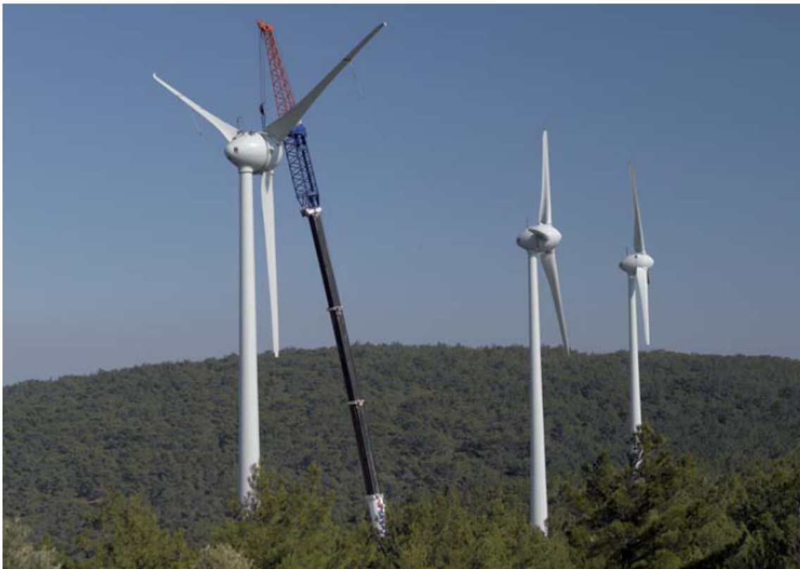
Manastir/West Turkey: First E-44 turbines in being installed in wind farm.
