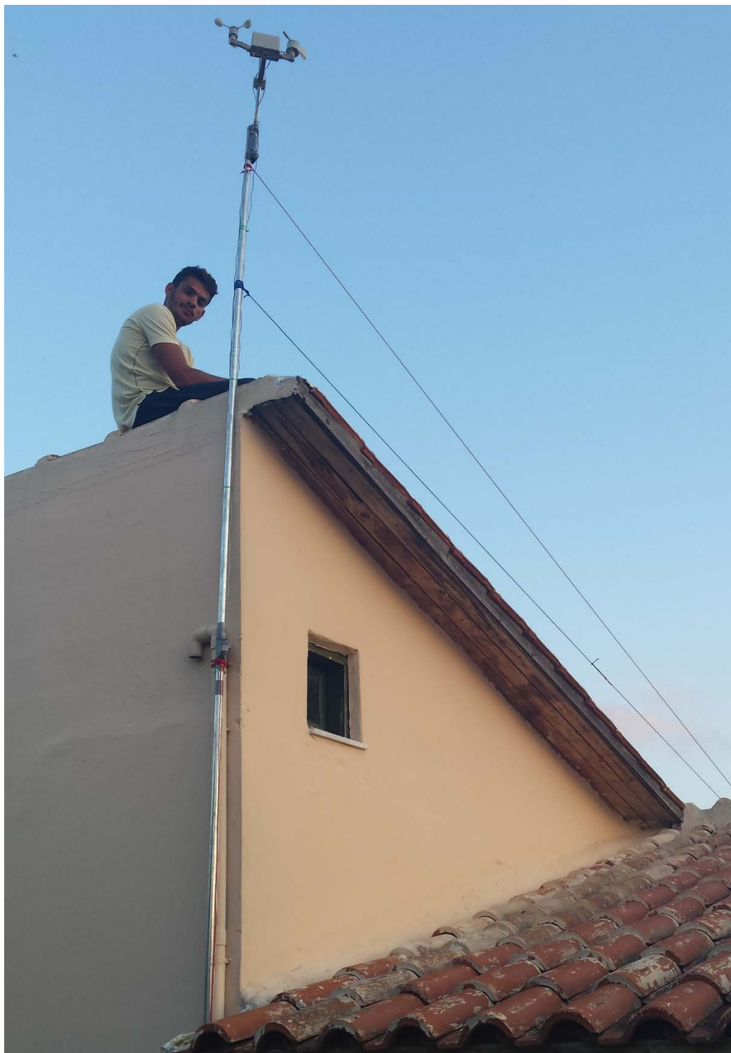
Figure 20 - The column in which the Weather Meters are mounted. My best friend Giorgos helped me to set up the column.
