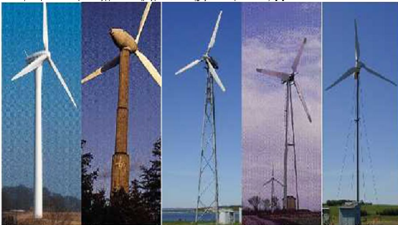
Tubular steel tower
