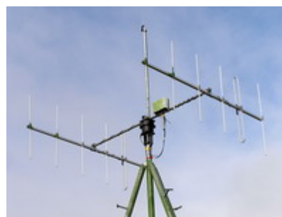
Close up of 6 element twin Yagi array ontop of a tower
