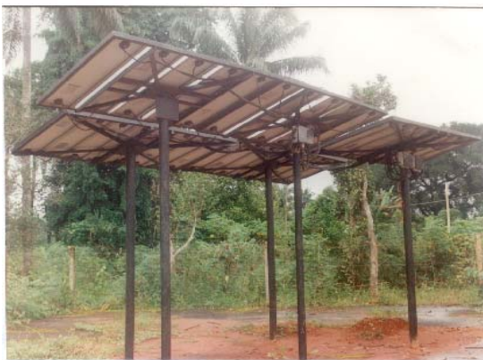
Figure. 12 1.87 kWp PV Village Electrification, Iheakpu-Awka, Enugu State FIGURE 11. Solar water heater
