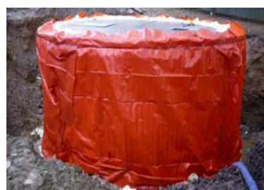
Tank 2 with a wrap of HD polyethylene
