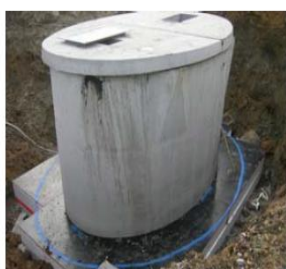
Tank 2 on 600mm insulation
