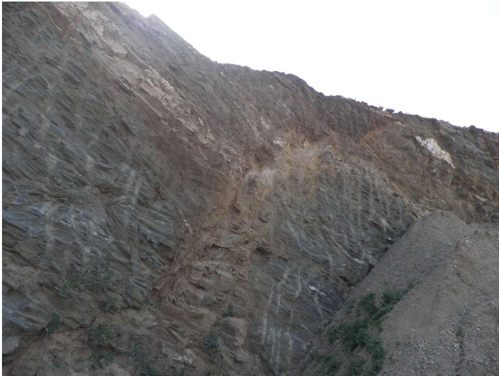
Normal geological fault
